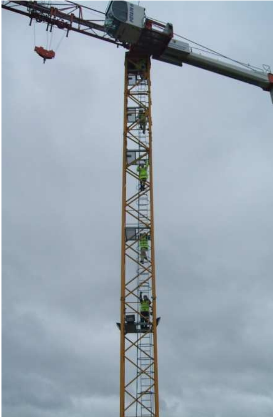
Climbing the crane
