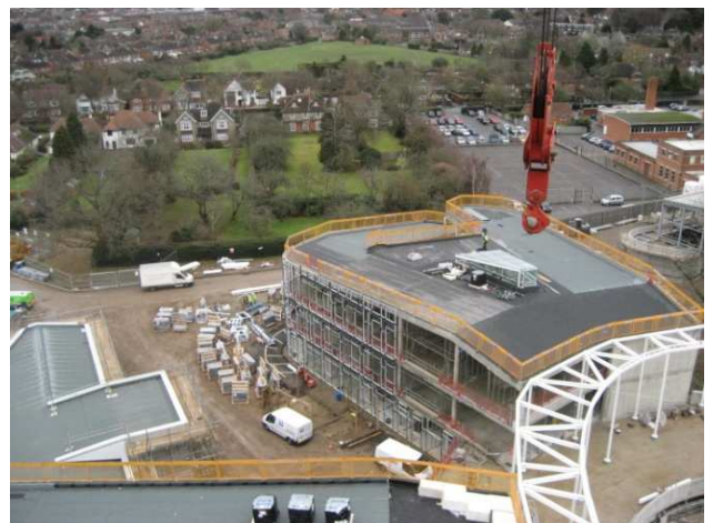
The new Wormestall block
